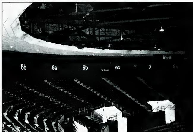
Figure 12. After acoustical modifications. Note the Helmholtz cylinders.
