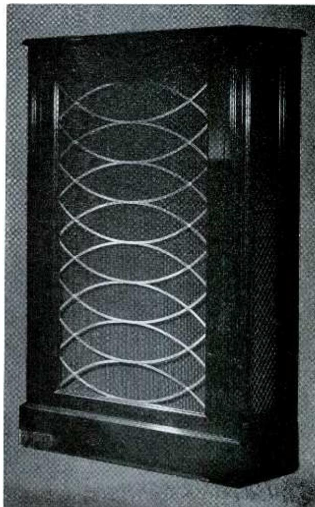
*This is one of the largest corner designs. It stands 5 ft. high and utilizes 5 speakers. Note that, unlike the other corner designs illustrated, the low frequencies do not radiate directly into the room. Sound from it is forced through a long, "horn" path.*
