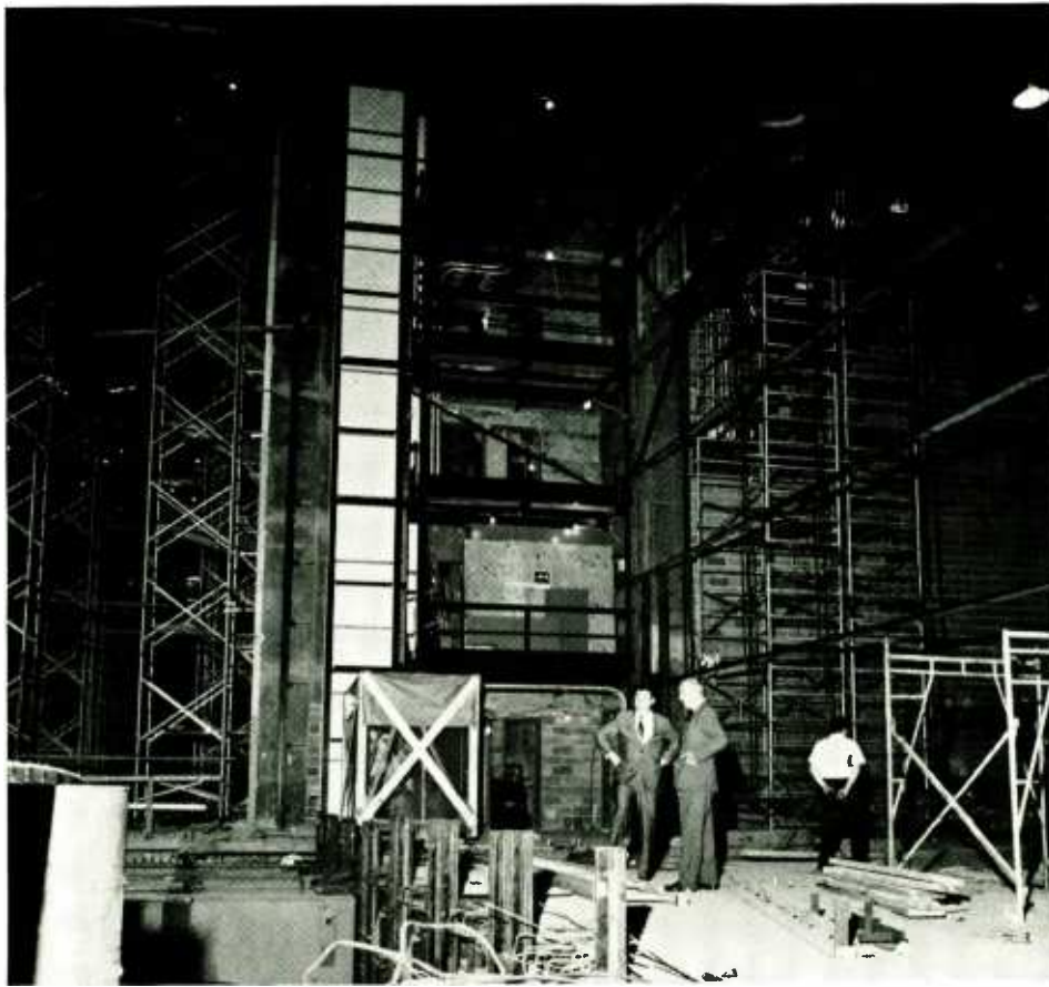
Scaffolding, cables, an open pit—the last to house the stage elevator platform.
