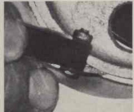
*Ampex brake band clearance check.*
