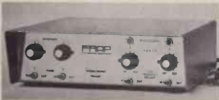
The output of the FRAP is transformer isolated low impedance and at microphone level, which necessitates returning at mike level or adding amplifiers which can be easily done with a number of good pre-amps available. Or, because the FRAP utilizes integrated circuitry it is possible to change the feedback loop of the final stage and have a line output, although a price will be paid in noise.
