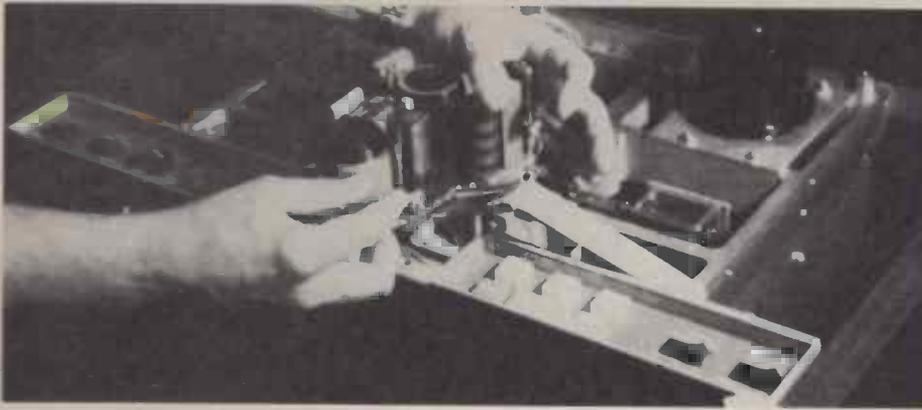
*3M pinch roller tilt adjustment.*
