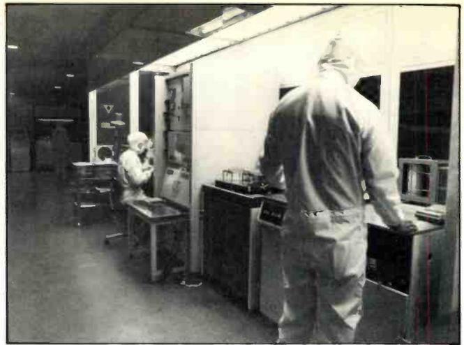
Glass Master preparation and photo-resist coating in the A-Room at Shizouka.
