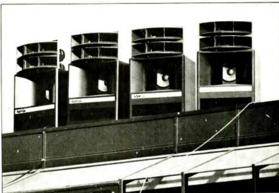
Figure 10: Roof-mounted RAMSA loudspeaker clusters at Pepperdine University's Raleigh Runnels Memorial Pool, where 5,000 spectators attended Olympics water polo events. The sound system was operated by the event commentators.
