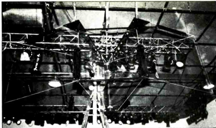
The main stereo array suspended in front of the Buddy Rich Band was fabricated from four, four-foot by four-foot sheets of plexiglass, with two Crown PZM-31 elements mounted in the top apex corners.
