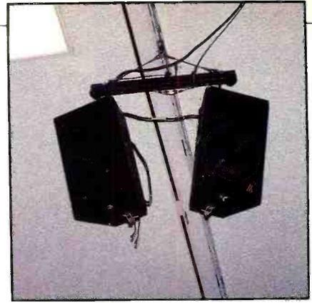
**Photo 10.** A pair of Meyer UPA-1A enclosures are easily suspended from simple hanging hardware in a low-ceiling ballroom. The UPA-1A is typical of the single 12-inch box with horn/driver components in a trapezoidal package, available from several manufacturers.
