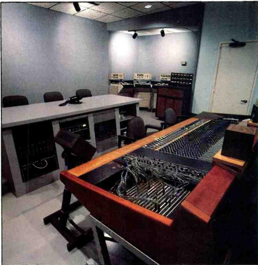
Each control room houses a Harrison 32 series console, MCI JH-24 machine, UREI 813 monitors tuned with White and UREI EQs, Auratones and a combination of Yamaha 2200 and UREI 6300 power amps.
