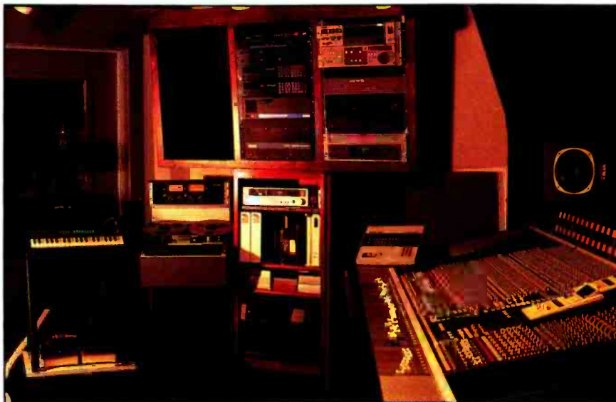
Studio B showing one of two outboard racks.
