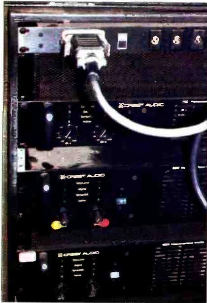
Figure 1. A custom "steering box" allowed the amp racks to be switched to the left or right mains without repatching.
