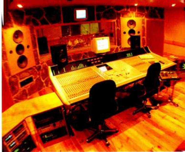
▲ Spain Music recording facility AreaMaster recently opened a new studio complex designed by renowned acoustician and Studio Sound contributor Philip Newell. The complex offers four day-lit rooms with air conditioning and a view over the surrounding mountains. Centre to the main room is a 40-channel D&R Octagon console with dynamics and moving faders. The second room houses a 32-channel D&R Orion console and the facility also offers three fully-equipped rehearsal rooms, bar area, private car park, satellite TV and an outdoor terrace.
