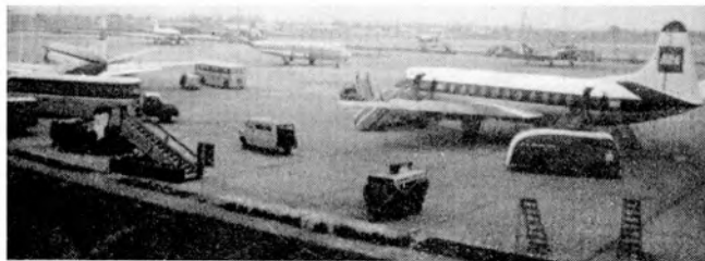
London Airport seen from the roof gardens.
