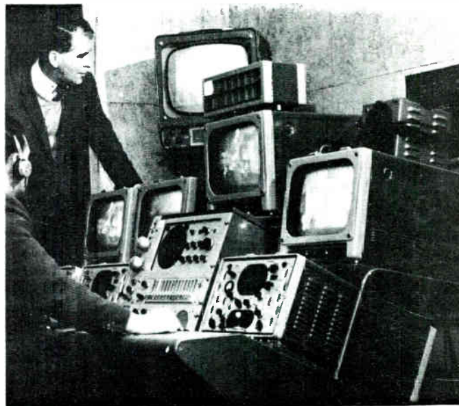
Studio A Control Room
