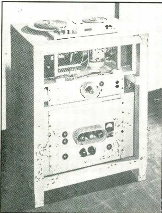
K4 Magnetophon (with hf bias)—date 1940.
