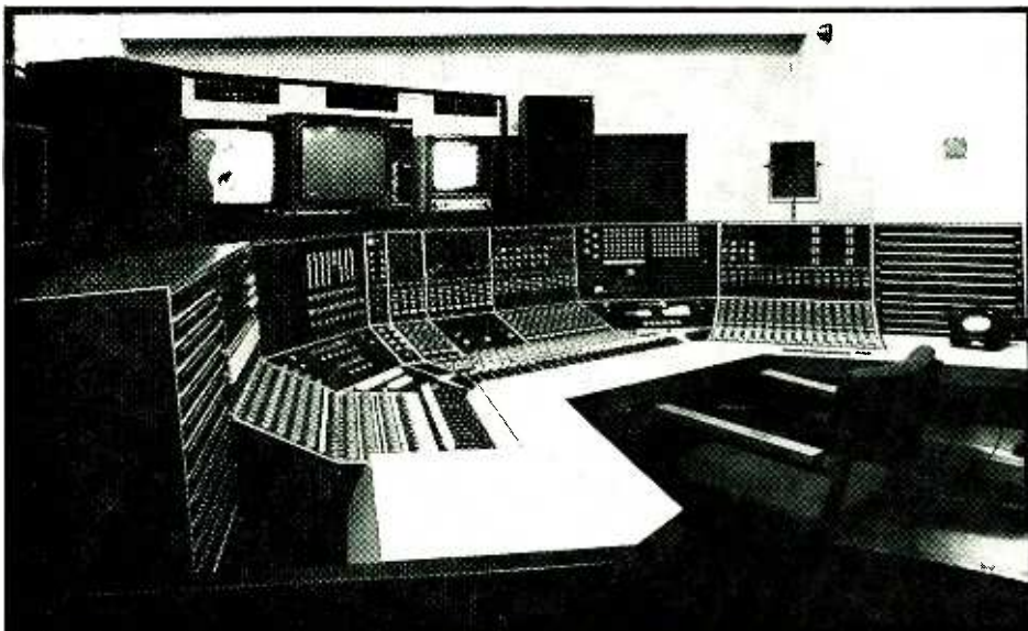
4418 Calrec desk installed last year at BBC tv studios, Glasgow.
