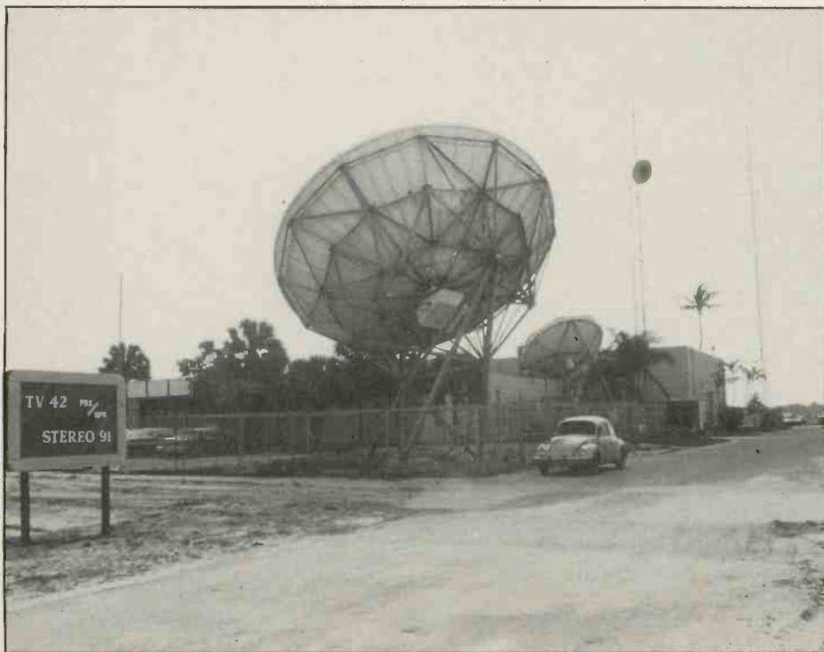
Antennas at NPR member station Stereo 91 (WHRF FM), Boynton Beach, Florida
