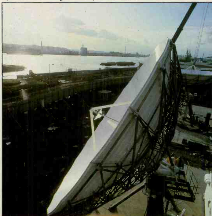
Uplink aerial working to ECS1 (photo: British Telecom)
