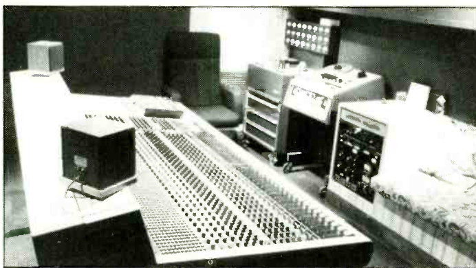
ICC Studio One control room with Trident Series 80 console
