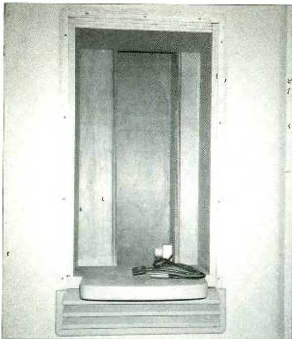
To compensate for the heat generated by the Genelec monitors, special ventilation chimneys were built into the back of each enclosure
