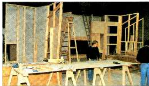
Modular studio construction at KFA
