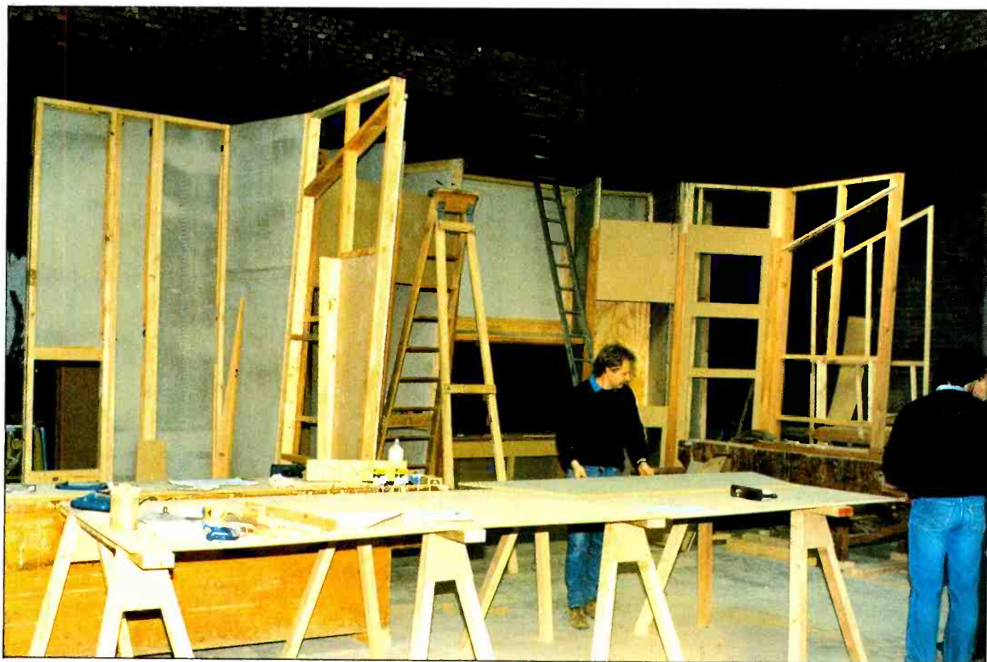
Studio construction using the modular approach at KFA's factory in London
