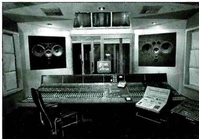
Neve VR60 installed at Orinoco, London
