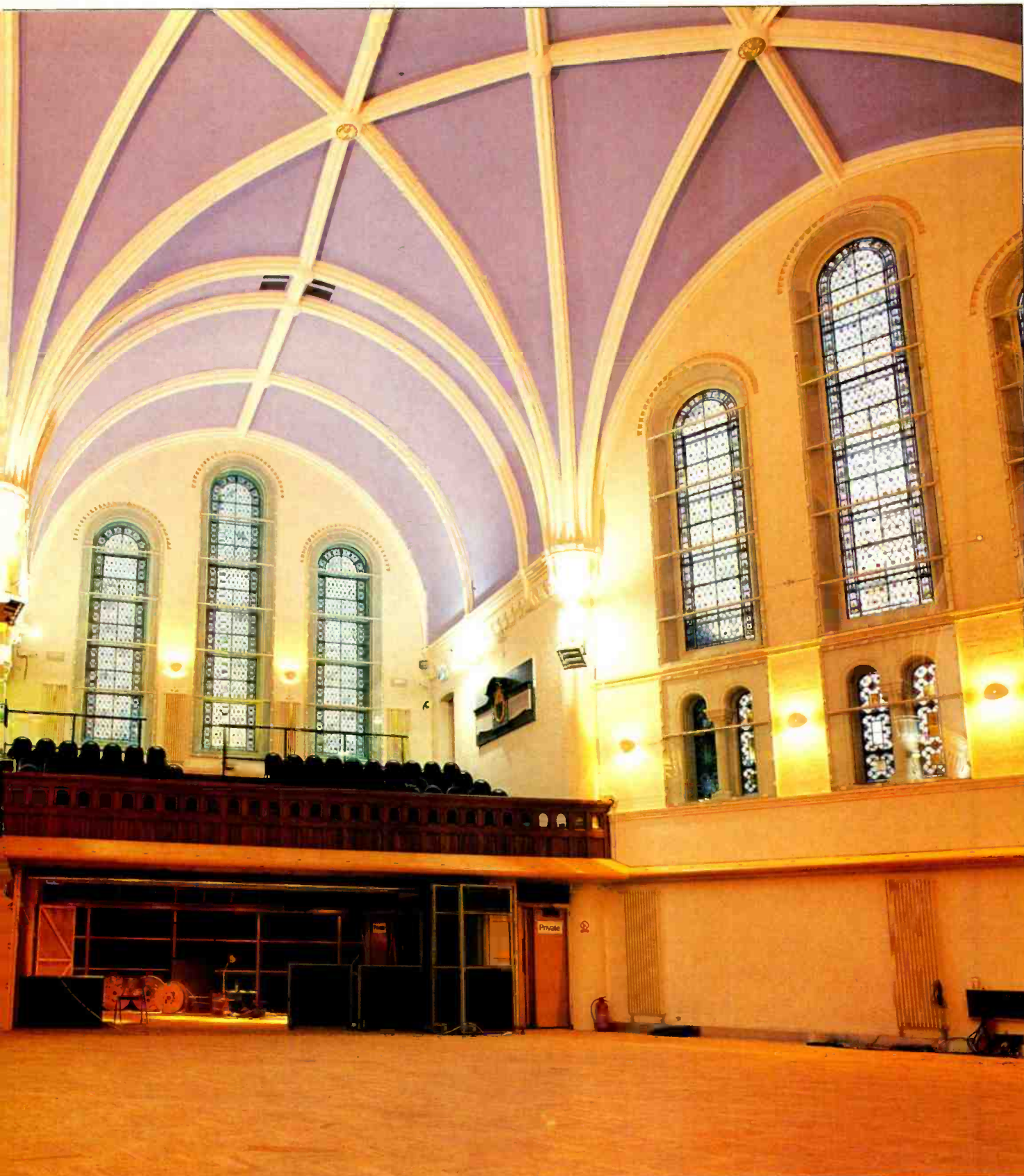
Air Lyndhurst's Main Hall nears completion
