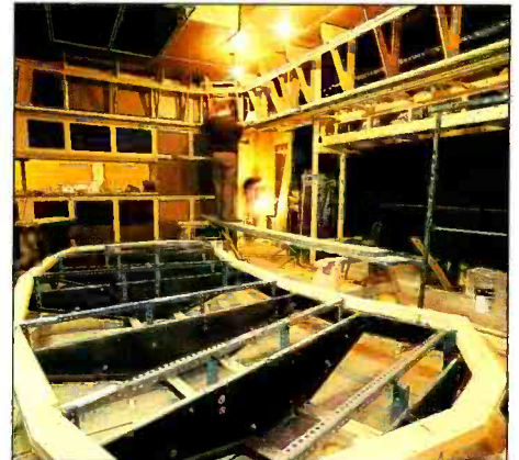
Studio 2 Control Room with 'acoustic cloud' on the floor awaiting fixture to the ceiling
