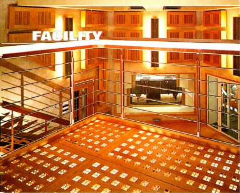
The view from the gallery showing RPG diffusers and plain plaster walls
