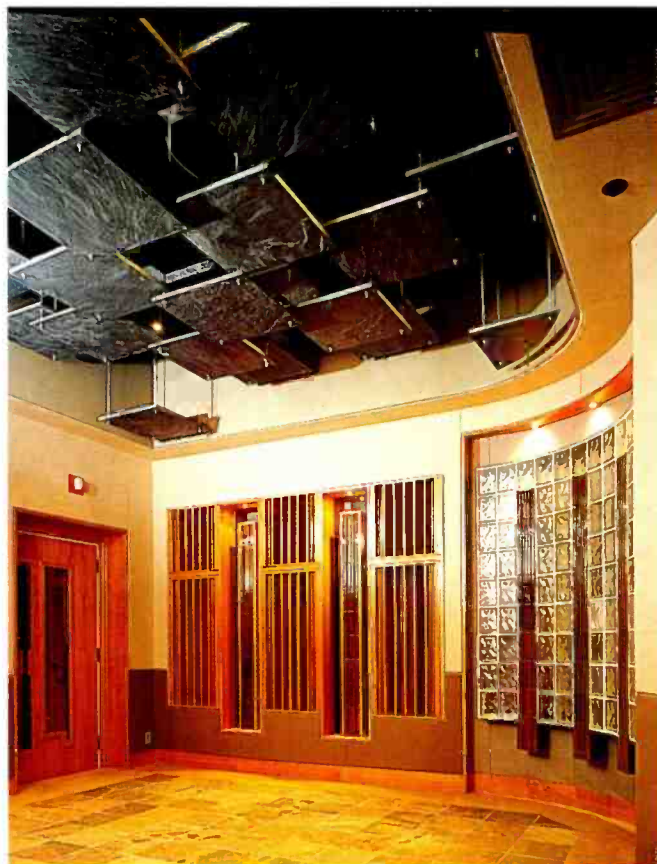
Quadratic series diffusers grace both the walls and ceiling in sections of both live areas
