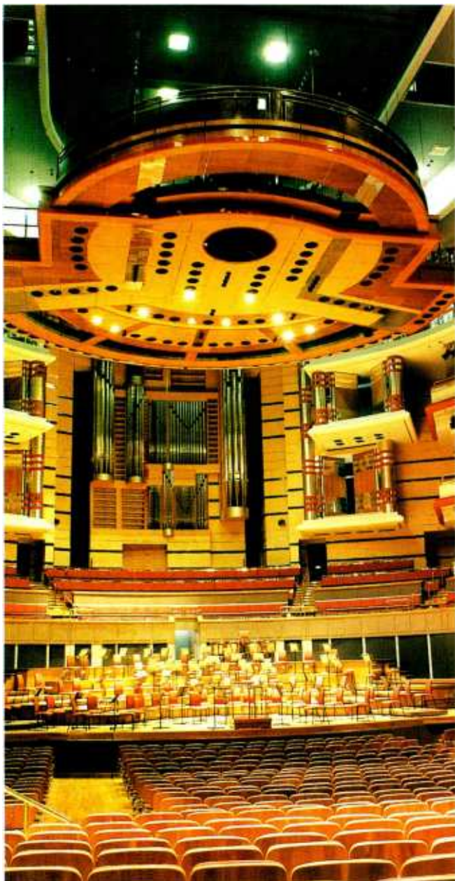
▲ UK: The acoustic hood in Birmingham's prestigious Symphony Hall has been improved in order to accommodate the increasing demands made on it by additional audio and lighting rigging. The 35-tonne hood that provides the principle means of controlling the auditorium acoustic is now suspended from 28 new cable assemblies designed by Midlands-based PCM, that incorporate strain gauged load link transformer capable of monitoring the load on the hood and an alarm facility. PCM, UK. Tel: +44 1226 864444
