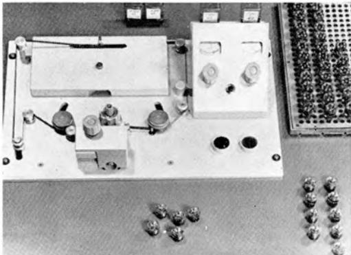
**Above left:** Six drilling operations, in Switzerland, means one operator and six drills. No time-consuming bit-changing.
