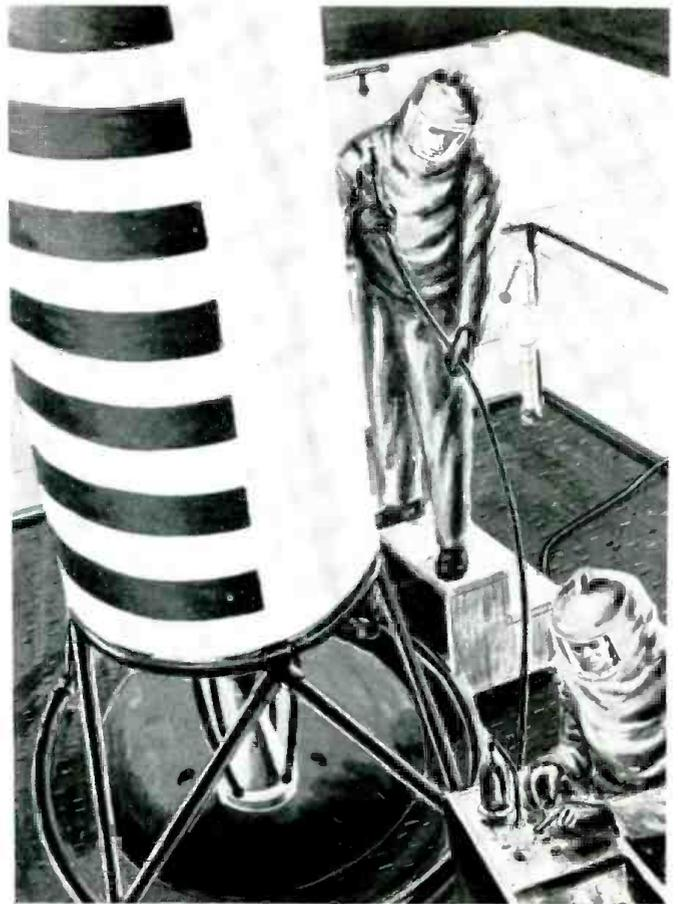
Left, the Vanguard rocket looks like a giant rifle bullet. Its payload will be a 20 inch sphere crammed with scientific instrumentation. To enter the orbit the satellite will have to obtain a velocity roughly ten times as great as that of a high powered rifle bullet. Right, fueling the rocket is a delicate task. Several of the liquids used in Vanguard are corrosive or inflammable and men must be dressed in protective clothing.
