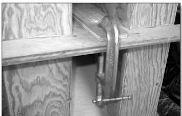
PHOTO 16: Installing the back brace.
