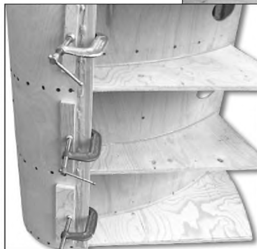
◀ PHOTO 16: Applying the back sheathing.
