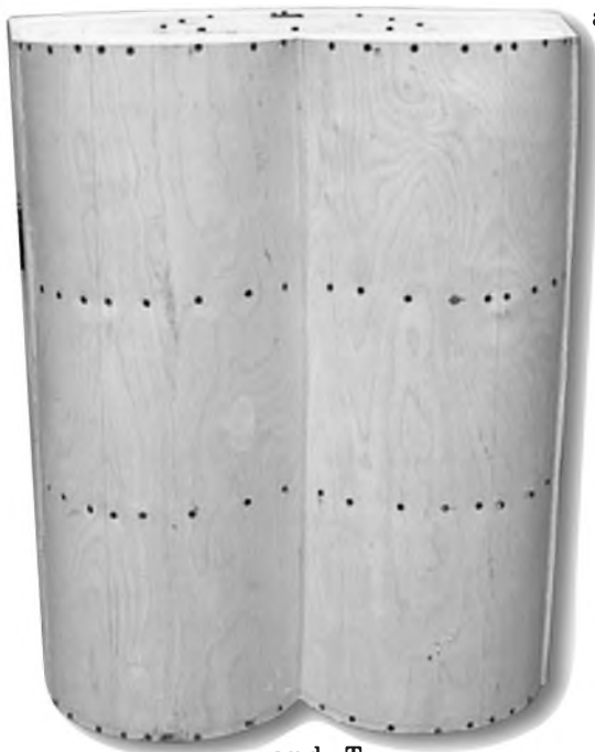
and T- PHOTO 17: Installing the sides.
