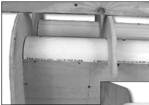
◀ PHOTO 13: Aligning back braces.
