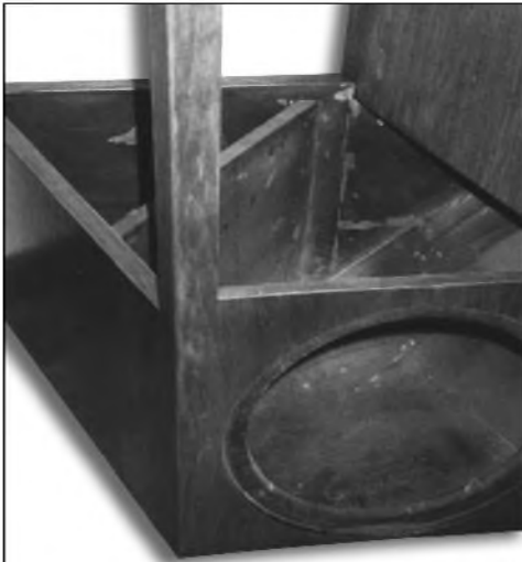
PHOTO 4: The woofer section of the TL with the top plate removed prior to final assembly.
