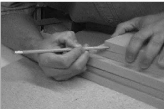
PHOTO 4: Marking the reference corner.
