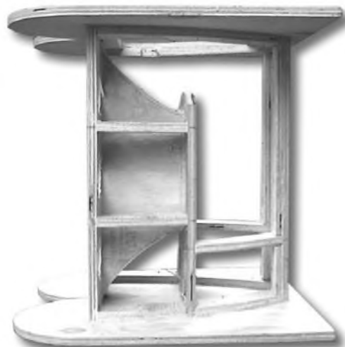
PHOTO 10: The assembly ready for sheathing.
