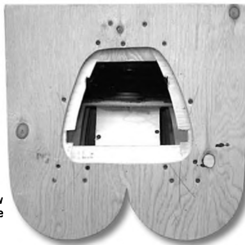
PHOTO 11: View through porthole after attaching the flanges.
