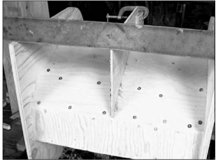
PHOTO 17: Truing the side braces with a straightedge.
