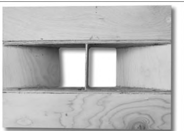
PHOTO 6: The throat horn attached to the horn supports.
