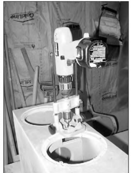
PHOTO 16: Drilling holes for the driver mounting T-nuts.
