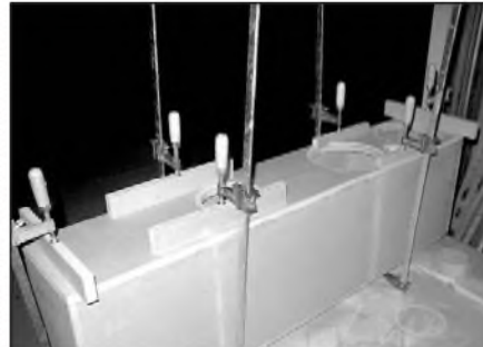
PHOTO 15: Gluing on the front. The back is done the same way.
