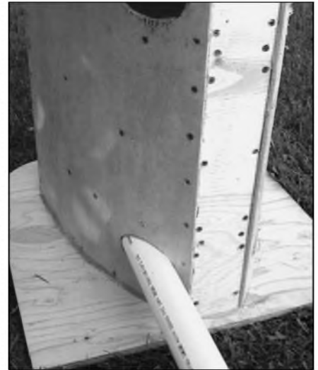
PHOTO 14: Checking duct hole for proper fit.
