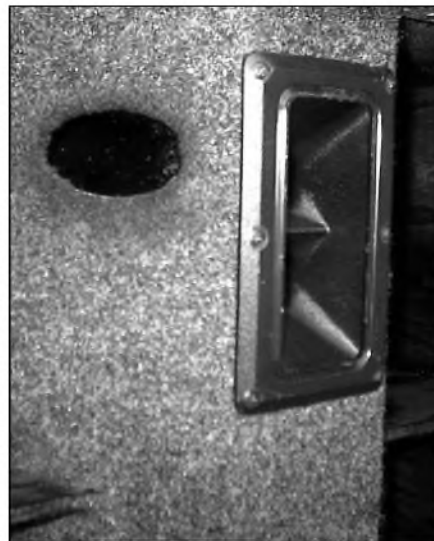
PHOTO 23: "Torpedo tube" duct on finished cabinet.
