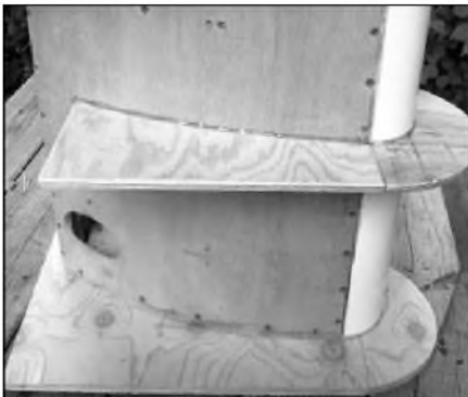
PHOTO 20: All bracing installed.
