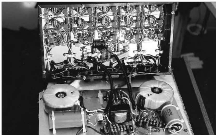
PHOTO 4: Power supply completed and connected into main chassis. Also note switch leads coming from barrier strips.
