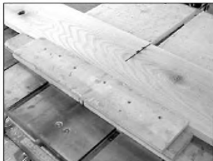
PHOTO 7: Cutting to length with a panel-cutting jig.
