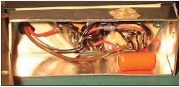
PHOTO 6: The simple oscillator circuitry is mounted under the 6KG6A socket.
