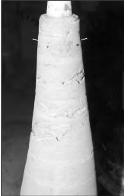
PHOTO 10: Patch up any blemishes on your concrete shell.
