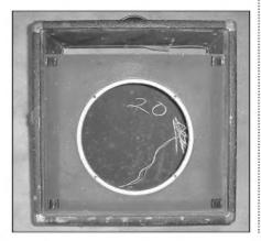
PHOTO 4: Enclosure routed for adapter ring.
