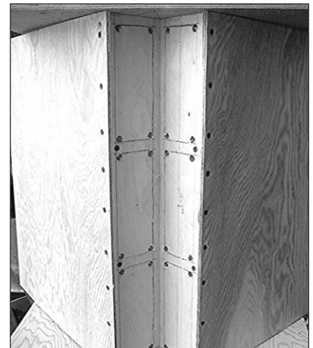
PHOTO 13: Beginning the sheathing of the horn.
