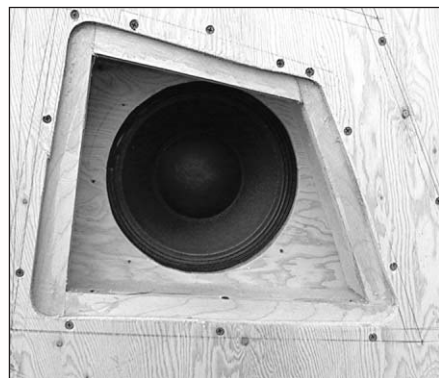
PHOTO 10: A porthole with flange installed.
