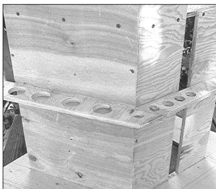
PHOTO 6: Attaching braces to the horn plates.
