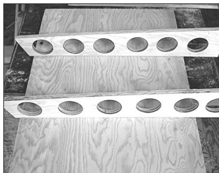
PHOTO 7: Attaching braces to a horn plate prior to plate installation.
