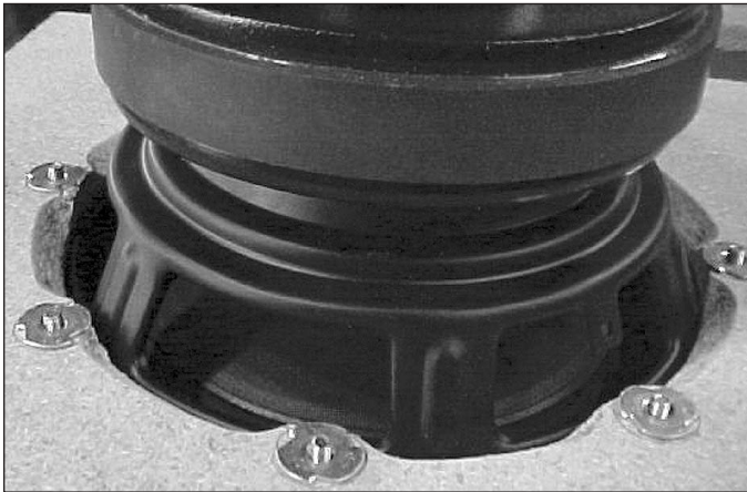
PHOTO 9: Rear view of front panel with driver mounted.
