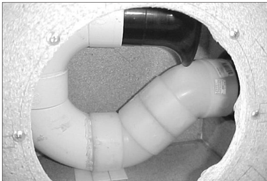
PHOTO 11: View of longer port structure through driver hole.
