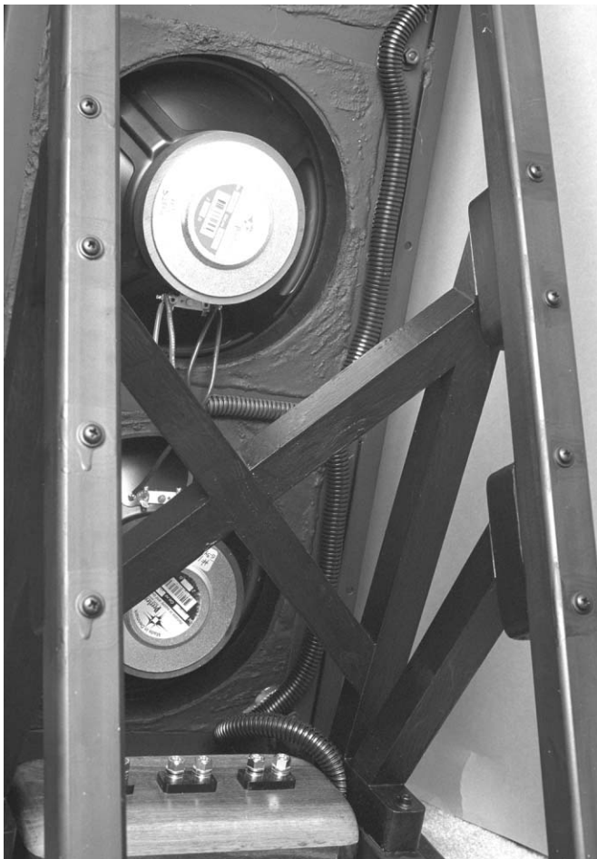
PHOTO 30: End view of brace.
