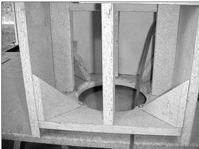
PHOTO 17: View inside box before installation of top.
