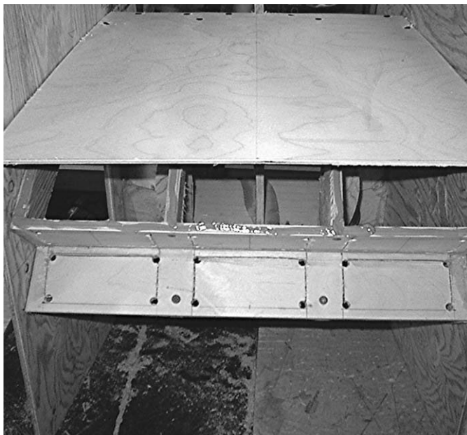
PHOTO 16: Installing the horn sheaths.
