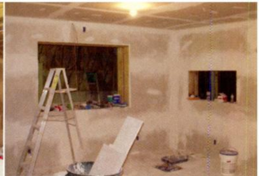
Room within a room construction: Sound Logic studios being built inside an old barn in the back yard. The photo at left shows the far wall to the control room being constructed. The middle photo shows the double wall design between the control and the tracking room. The photo at right shows the future control room, complete with two layers of sheetrock on each wall for solid soundproofing.
