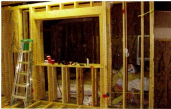
Room within a room construction: Sound Logic studios being built inside an old barn in the back yard. The photo at left shows the far wall to the control room being constructed. The middle photo shows the double wall design between the control and the tracking room. The photo at right shows the future control room, complete with two layers of sheetrock on each wall for solid soundproofing.
