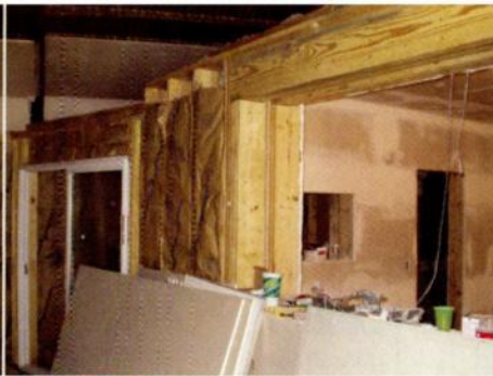
Room within a room construction: Sound Logic studios being built inside an old barn in the back yard. The photo at left shows the far wall to the control room being constructed. The middle photo shows the double wall design between the control and the tracking room. The photo at right shows the future control room, complete with two layers of sheetrock on each wall for solid soundproofing.
