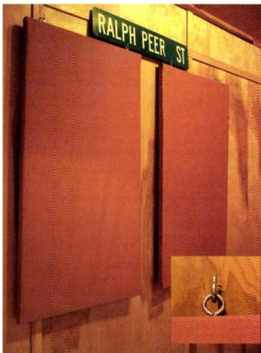
Fig. 2: You can attach acoustic treatment to a wall with hooks (see inset) so it’s easy to detach and reattach. This also makes any panels easy to flip around if you have a different type of treatment on the other side, thus giving you two types of treatment with one panel.
