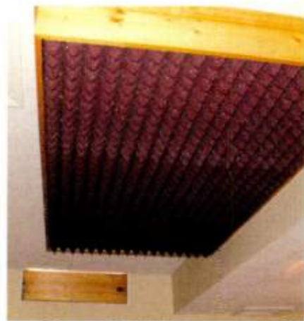
A small absorption canopy on a low ceiling can be effective at keeping early reflections from causing phase issues.
