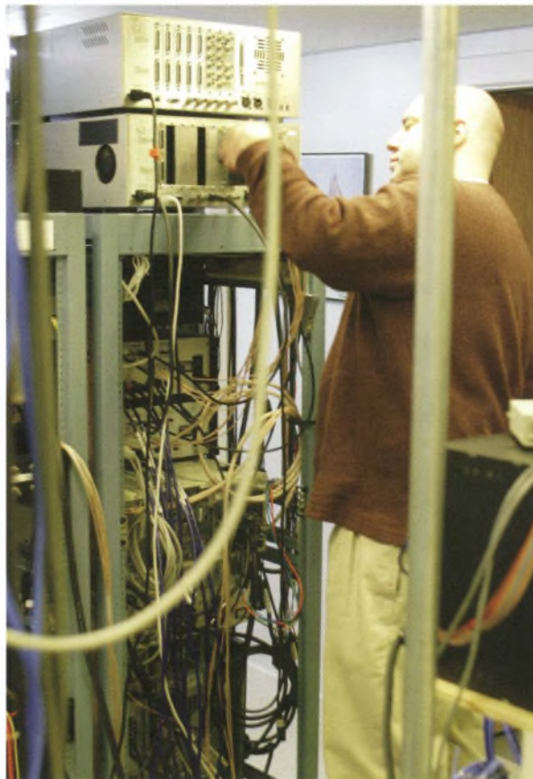
Mark Donahue checking connections.
