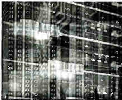
um cleaner hose directly over the top of gear, especially the console, and lift it from section to section so you don't knock dirt into crevices as you move. Small air filtration devices placed near equipment, especially down near the bottoms of racks, also help keep dust under control.
