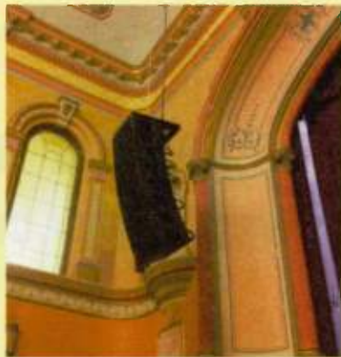
A new Adamson Metrix-I line array system with Metrix Sub-I dual 15-inch subwoofers was installed at Town Hall in Hawthorne, Australia.
