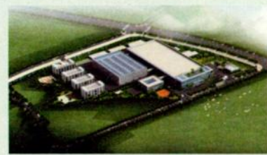
An artist's rendering of Music Group City, scheduled for completion in mid-2014.
