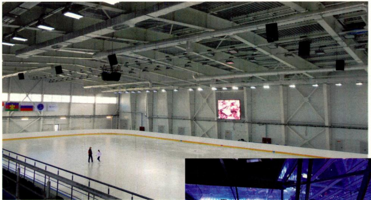
Training centers for hockey and figure skating were outfitted with multiple Renkus-Heinz TRX151 two-way systems.
