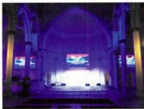
A half-dozen Renkus-Heinz VARIA VAX101 cabinets hang per side inside Oakland’s New Birth Church.
