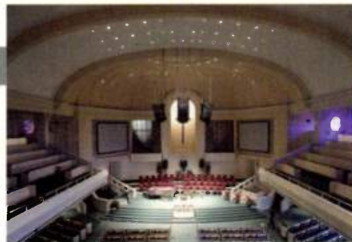
The installation of a Bose RoomMatch system at Lawton, OK's First Baptist Church marks use of Bose products on a Dante network.
