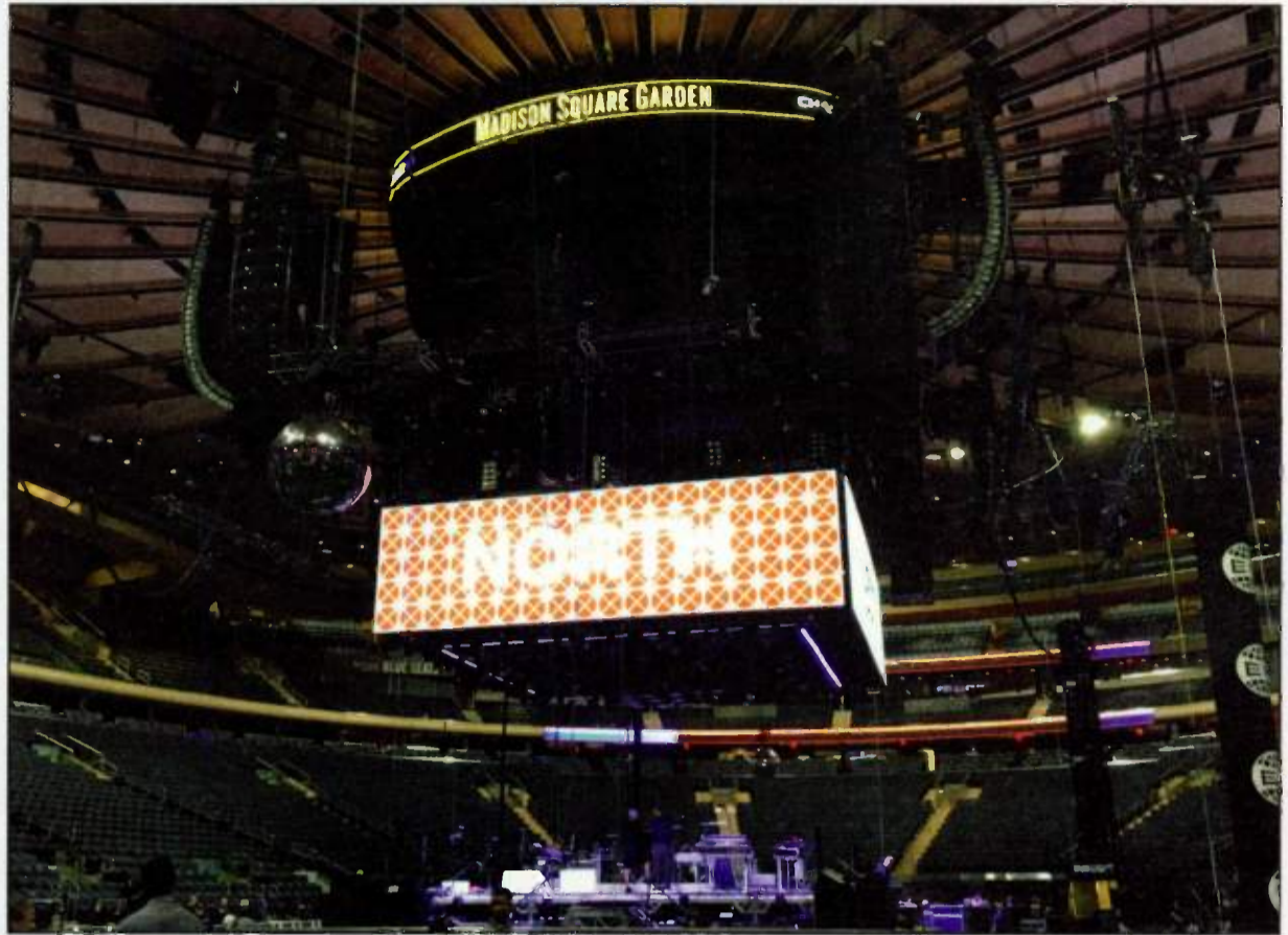
The massive L-Acoustics K1/K2 rig supplied by Solotech for Arcade Fire's tour is believed to be the largest AVB-based touring system yet assembled.
